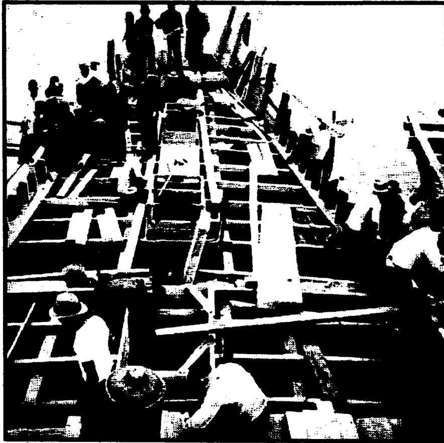
Figure 61: Numerous frames or chuanlei gu extended beyond the deck level in this image of the Sea Dragon under construction, Kowloon, China. (Halliburton, Halliburton, 386)
